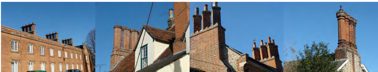
Selection of chimneys on listed buildings
