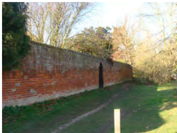
Picture 1.45 Prominent wall enclosing modern properties at Gibson Gardens. Walls both listed and unlisted are a particularly important feature in the conservation area
