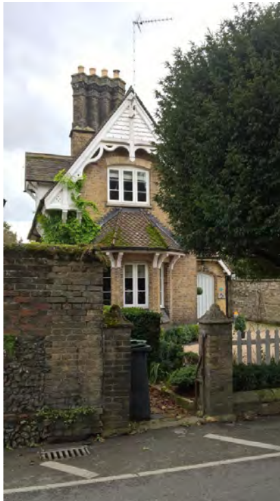
Picture 1.21 Elm Grove Lodge, Audley Road showing unusual gable bargeboard detailing,
