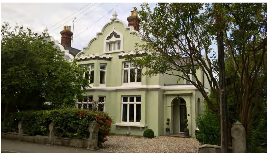
Picture 1.49 No 4 Mount Pleasant Road, one of a pair of exceptionally well detailed 19th century villas, forming part of a grouping along Mount Pleasant Road
