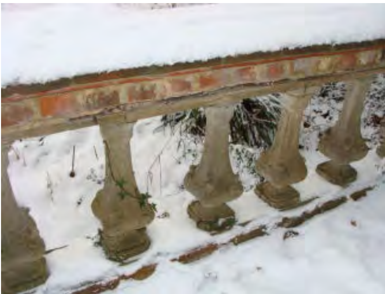
Picture 1.9 Fine 19th century boundary wall at Bridge End Garden
