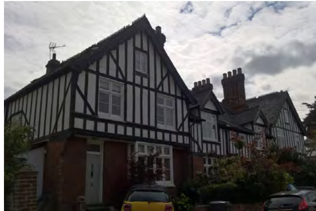
Picture 1.51 No.s 39 - 45 West Road, a terrace of two storey houses dating from the late 19th century with exquisite detailing including pargetting, decorative bargeboards and prominent brick chimney stacks.
